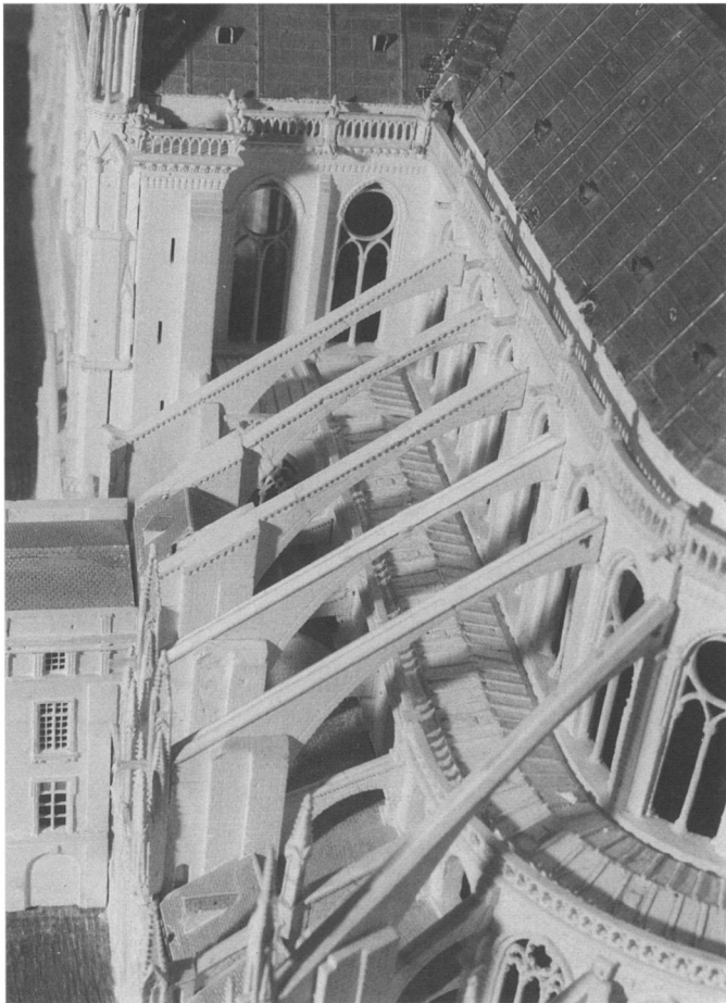
25 Plaster model of Notre-Dame, detail of south side flyers with chevron (photo: Murray)
